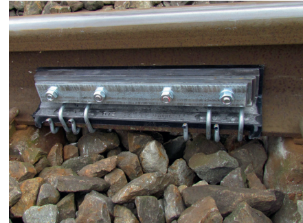
Tuned Dampers assembled on ballast track
